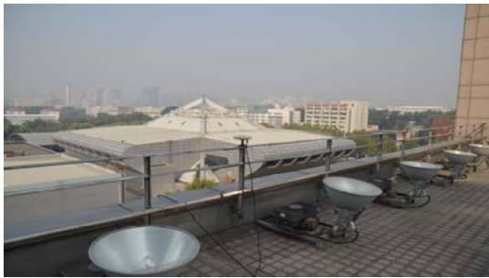
Figure 7. The Roof Top Where the Antenna is
